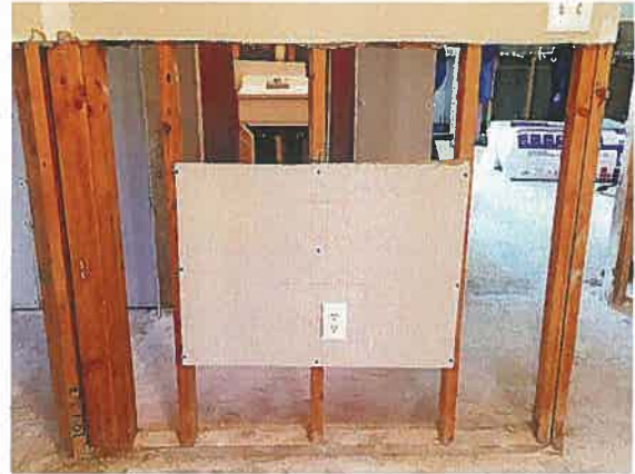
The contractor will make sure the electrical system is safe and working. This patch of drywall with the electrical outlet is temporary but functional.
